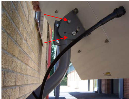
Figure 27 - Adjusting elevation
